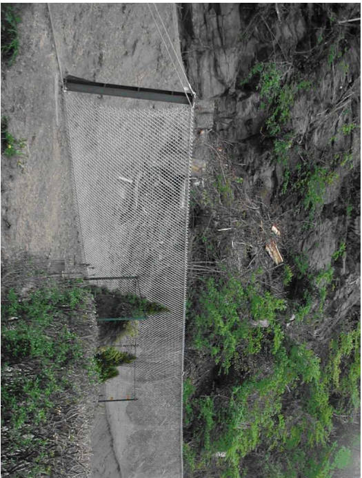
100kJ Rockfall Barrier without upslope anchors
